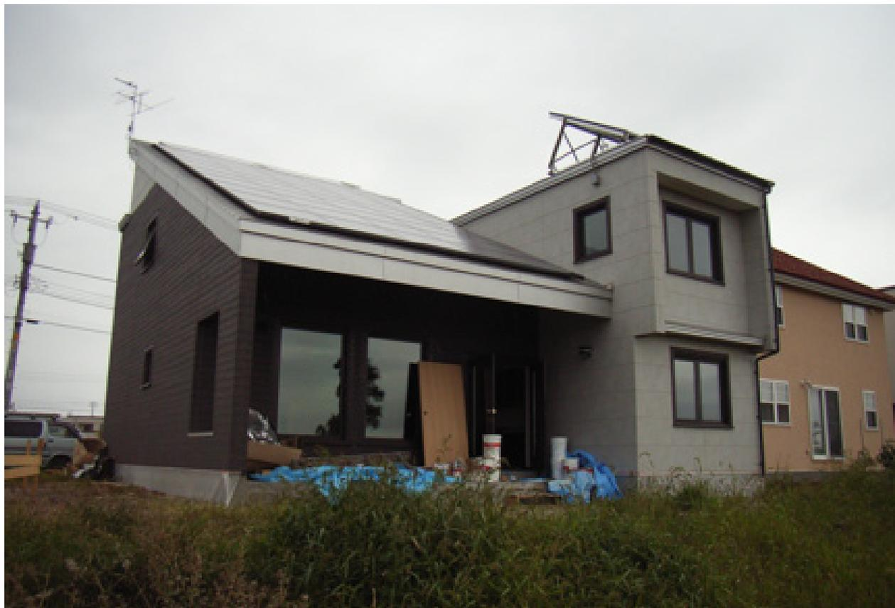
**The Sapporo net-zero energy house nearing completion. The large solar panels in the foreground generate about 7,600 kWh of electricity per year. The raised solar panel on the right is for heating domestic water.**
