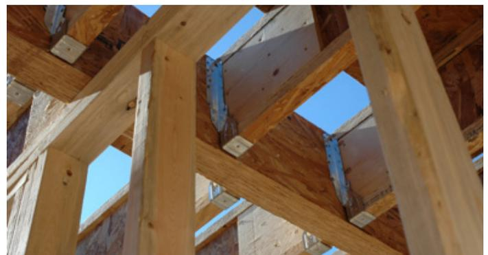
**Detail of the framing work. Note the use of I-joists, engineered framing using OSB rather than traditional solid lumber. The engineered beams are not only straighter and stronger than dimensional lumber, they are much more environmentally responsible.**
